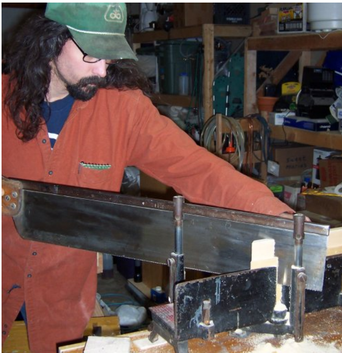
sawing the baseboard miters
